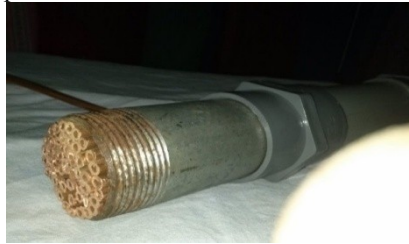
Figure 15. Copper tubes of hot heat exchanger
