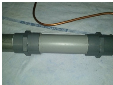
Figure: Stack enclosed by a PVC tube
