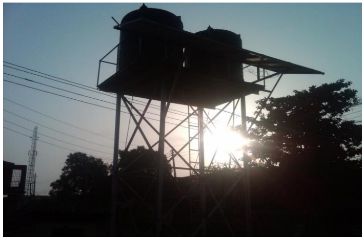
Plate 7: Solar Electric Pump Borehole at Uso Owo.
