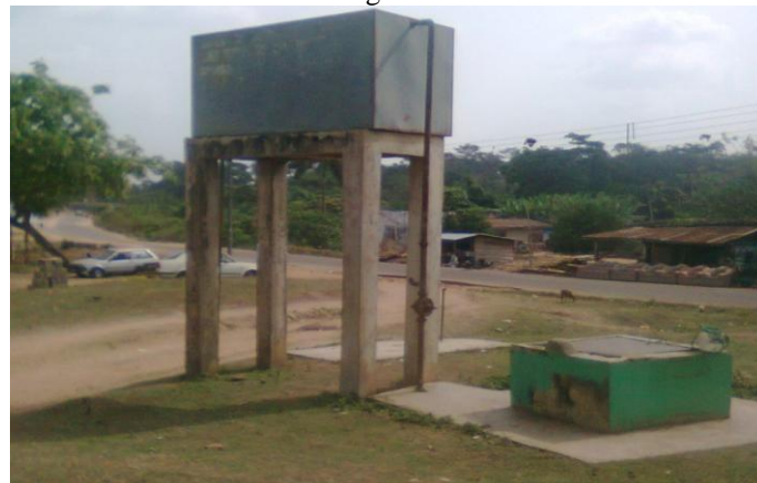
Plate 5: Electric Pump borehole at Idasen Owo
