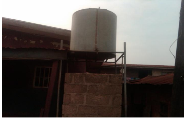
Plate 6: Electric Pump borehole in residential house at Ipemen Owo
