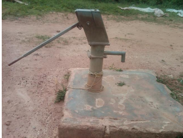
Plate 3: Hand Pump Borehole at Ipele Owo.
