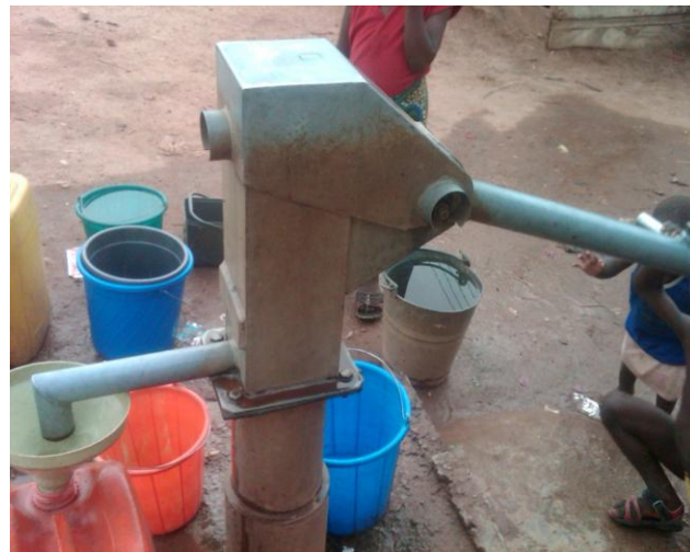
Plate 4: Hand Pump Borehole at Amurin
