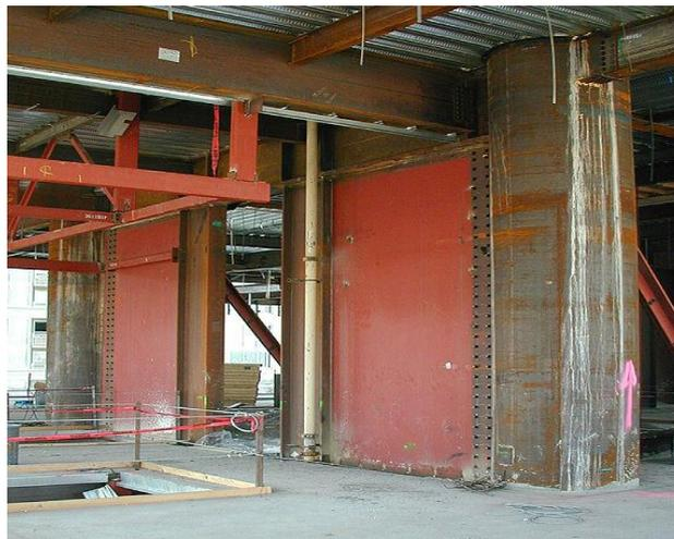
Figure 1. Coupled steel plate shear wall [1]
