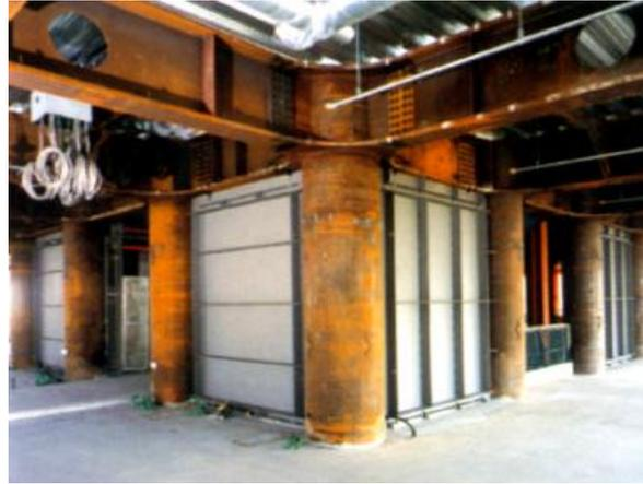
Figure 2. A view of building with steel plate shear walls and a close-up of the walls [1]
