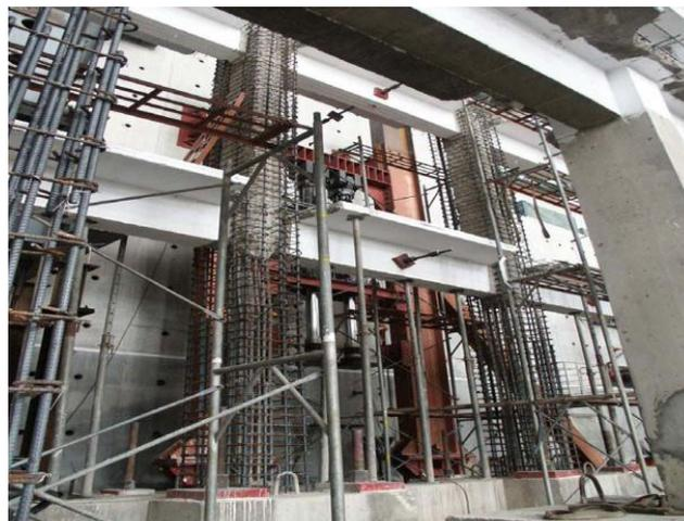
**Figure 18.** Retrofitting with RC Column Jacketing [12]
