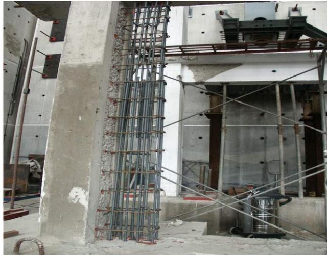
**Figure 16.** Retrofitted with RC Wing Wall
