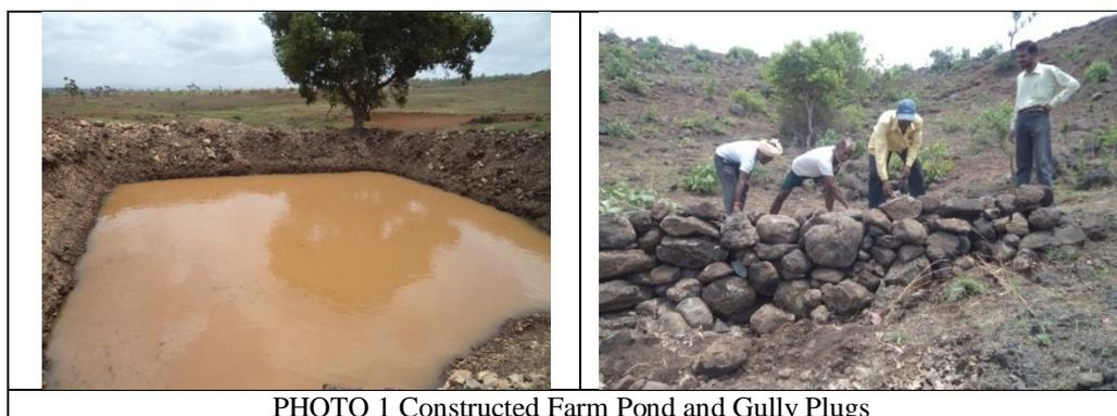
PHOTO 1 Constructed Farm Pond and Gully Plugs
