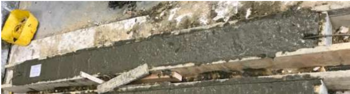
(a) Boreholes have been kept open during casting
