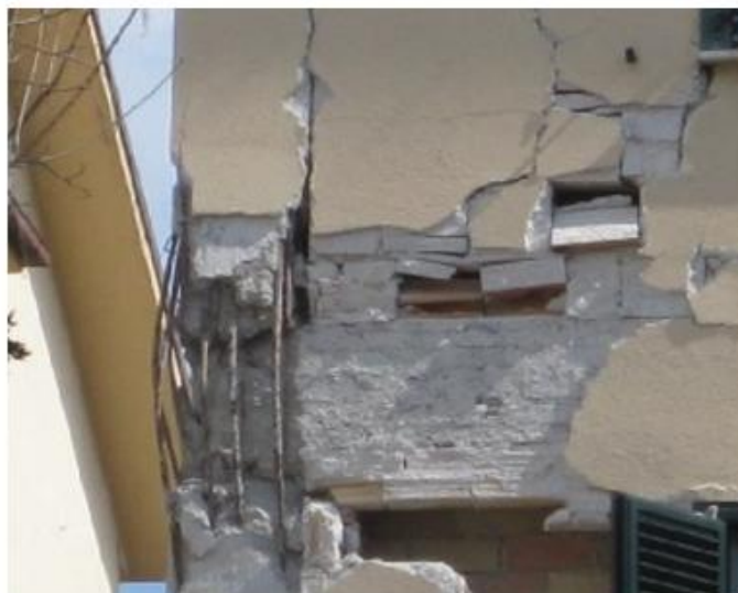
Figure no 1: Beam-column joints failures in Izmit earthquake in Turkey
