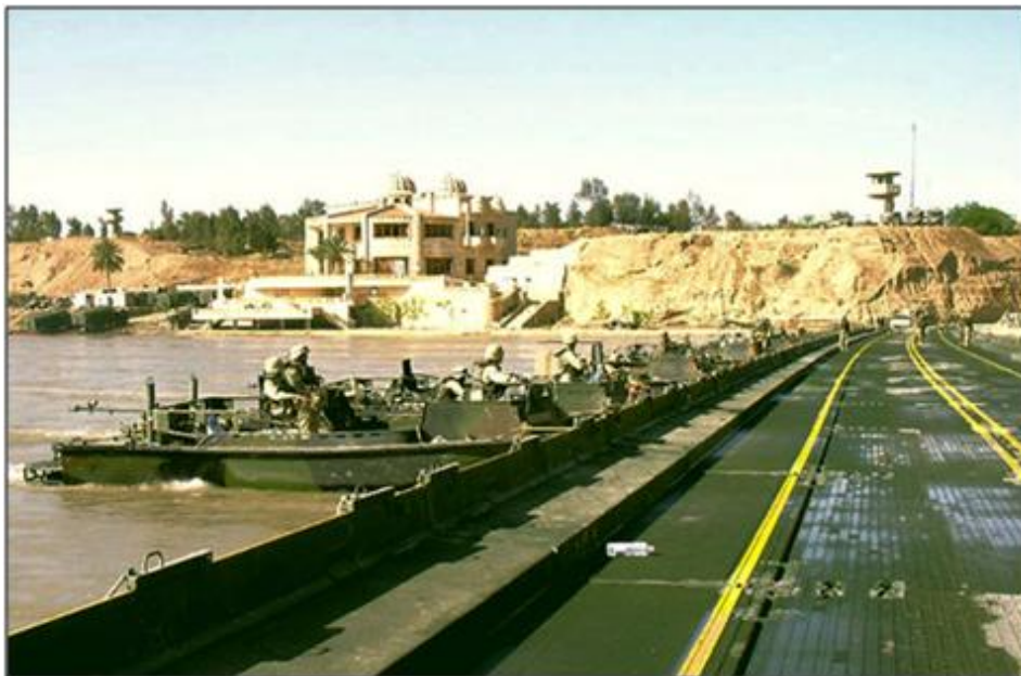
Figure 2. Photo of Pontoon bridge after installation over waterway
