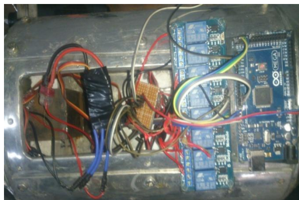
Fig. 14 Setup of control panel
