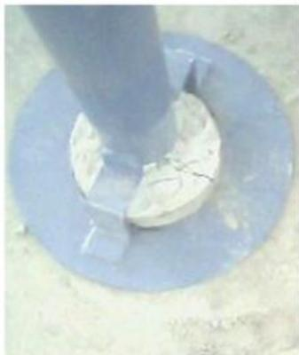
Fig.9 crack at initial stage
