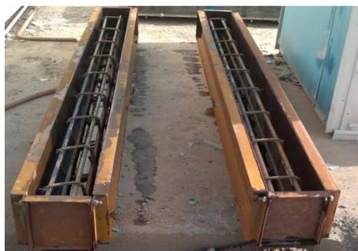
**Photo (1)** Steel moulds for casting the all reinforced concrete beams.
