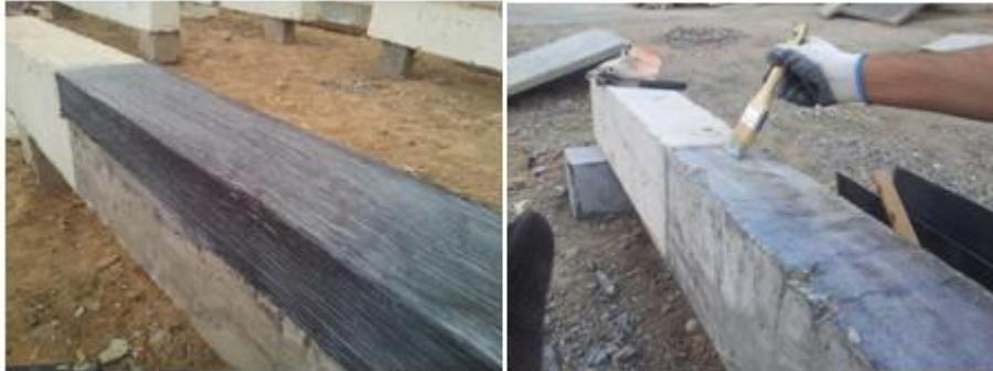
Photo (5) Method of rehabilitate the damaged beam using carbon fiber.
