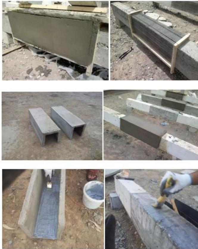
Photo (4) Methods of casting and fixing the ferrocement sections.
