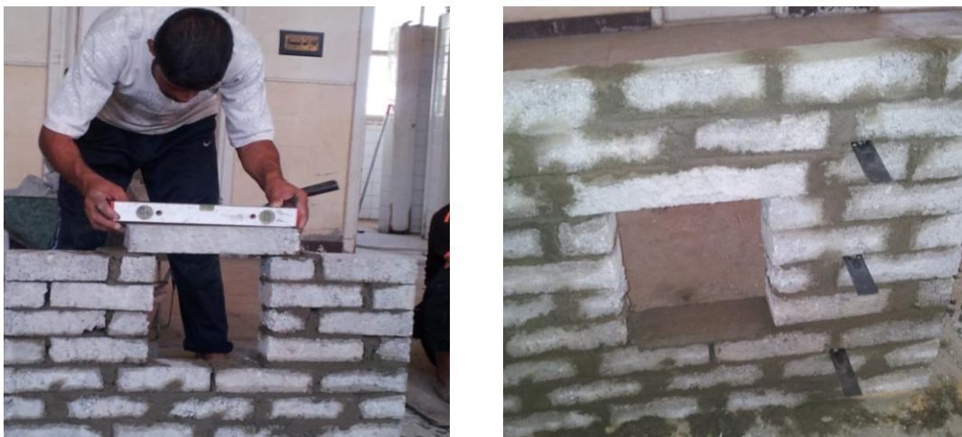
Fig- 3 Brick wall specimen during construction
