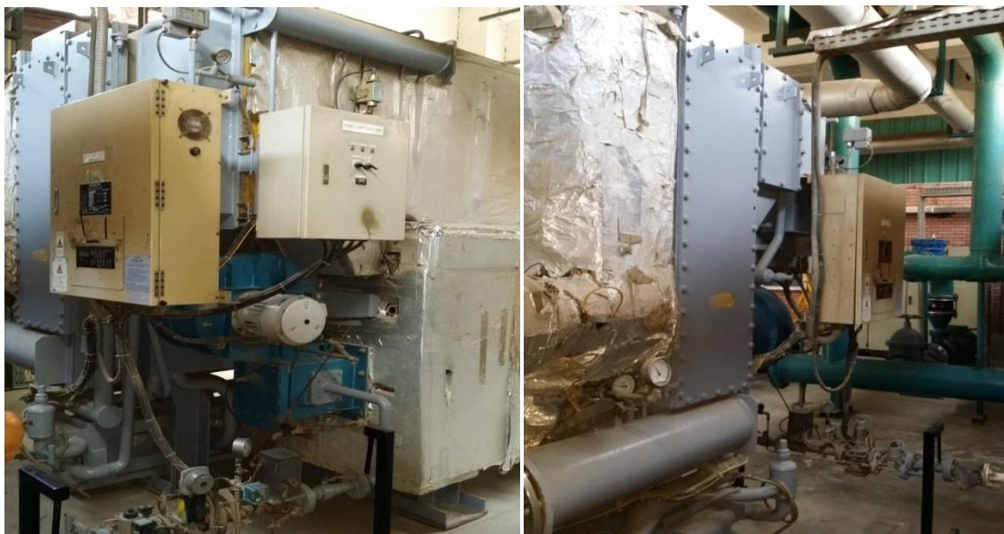
Fig.1. Parallel-flow double-effect absorption chiller view.
