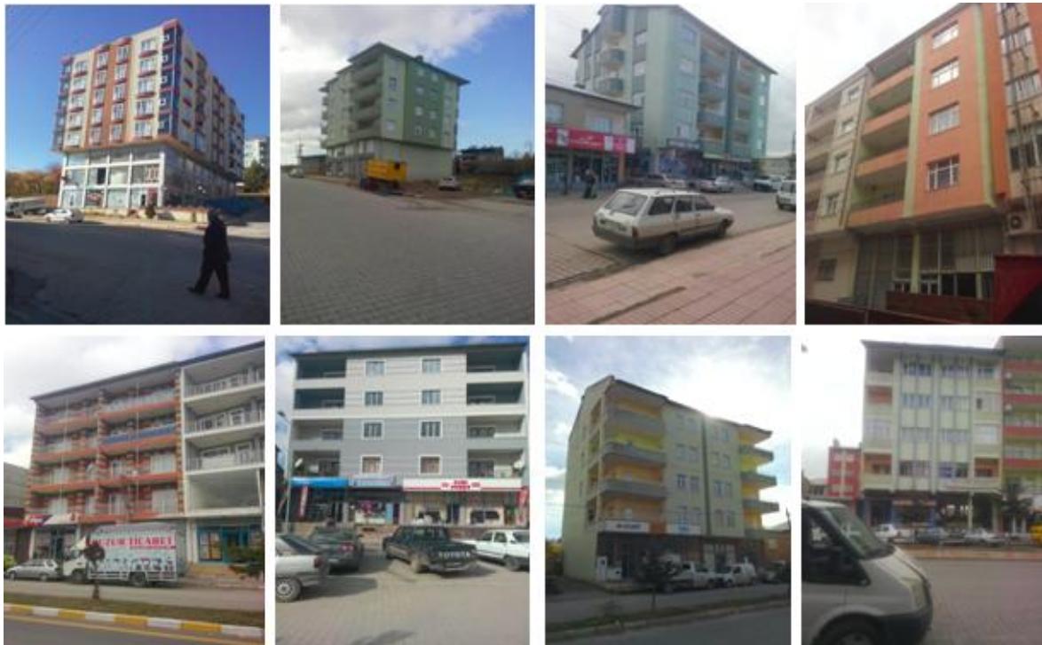
Fig. 4.1. Some pictures of investigated buildings
