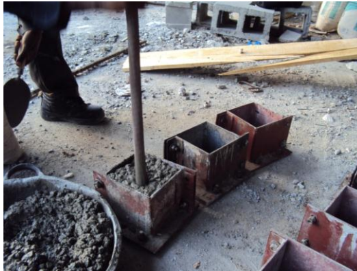
Plate 4: Compaction of fresh concrete with tapping rod
