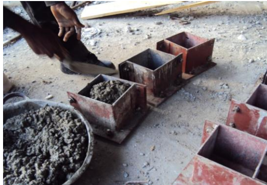
Plate 3: Casting of the concrete cubes
