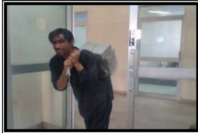
Fig.2. Extra load of building blocks carrying by labor (SSUET Site)
