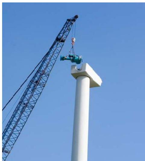
Fig 2.-Wind Turbine Gearbox Installation
