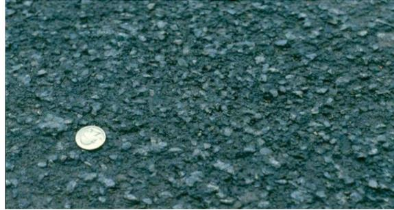
**Fig 12. High severity raveling of asphalt surface**
