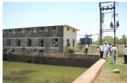
Fig. 6 No Desilting Done
