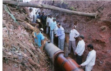
Fig 9 and Fig 10 Lowering Down of Invert Level of Existing Psc Raising Main and Installation of the same
