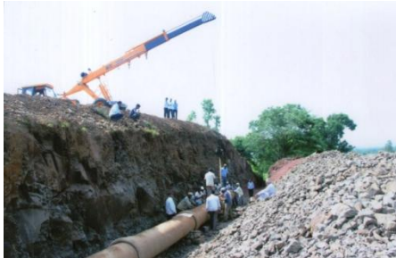
Fig 9 and Fig 10 Lowering Down of Invert Level of Existing Psc Raising Main and Installation of the same
