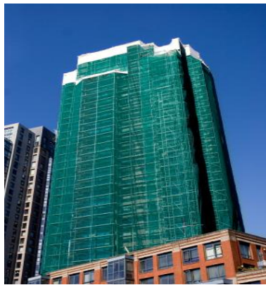
Fig. 1 Typical scaffolds surrounded by net
