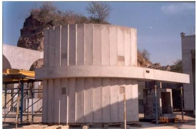
Photo.5. Mockup of single piece of precast canopy difficult to handle
