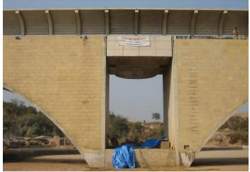
Photo.3. Independent slab separating two arch bridges
