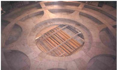
Photo.9. Provision of very irregular pattern of beams due to central opening
