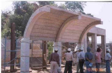
Photo.6. Mockup of three pieces of precast canopy to simplifying handling
