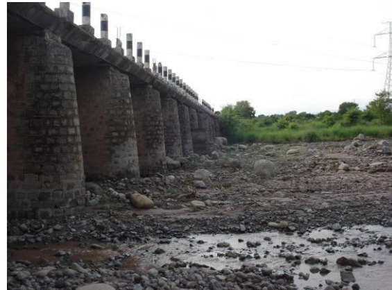
Photo.14. U/S side of bridge near km49 of NH21A
