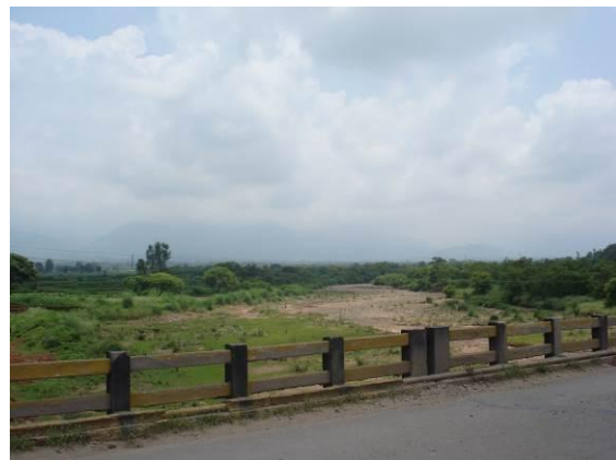
Photo.10. U/S side of bridge near km24 of NH21A
