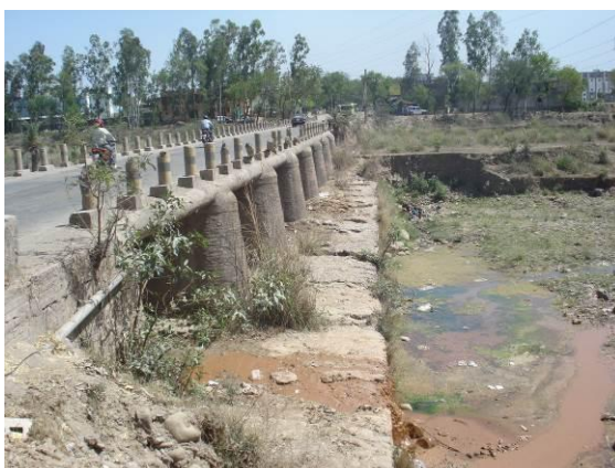
Photo.17. D/S side of bridge near km55 of NH21A
