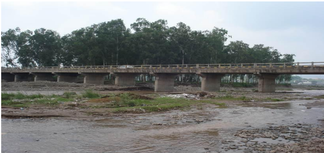
Photo.3. Presence of densely spaced trees on the upstream side
