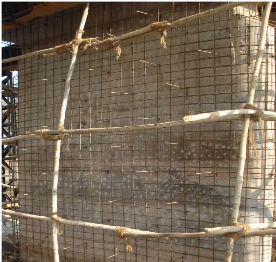
Photo.20. Concrete jacketing of pier and pier cap
