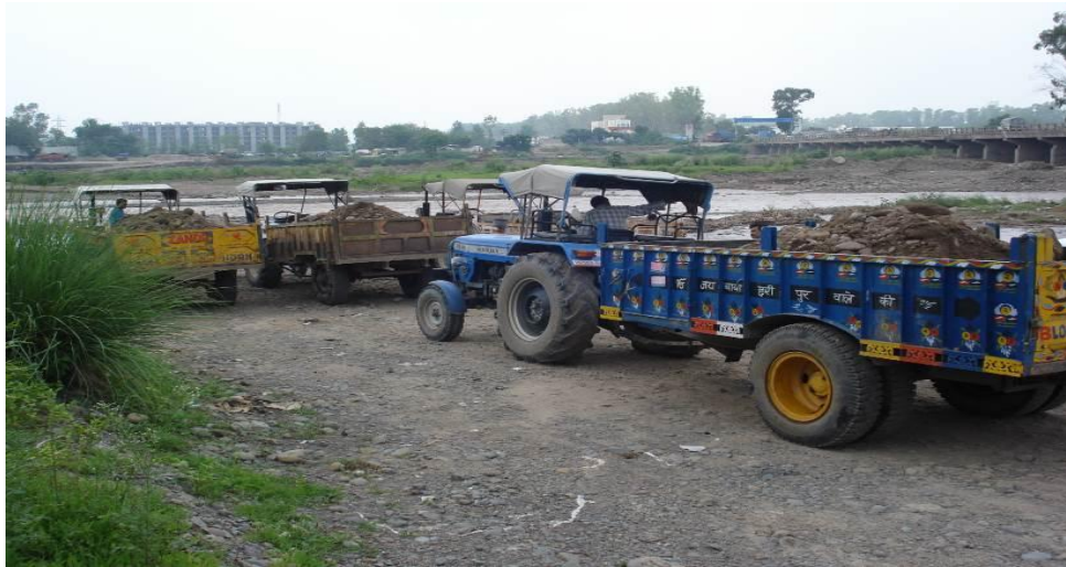
Photo.4. Mining taking place adjacent to the bridge site
