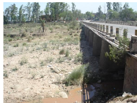
Photo.18. U/S side of bridge near km55 of NH21A
