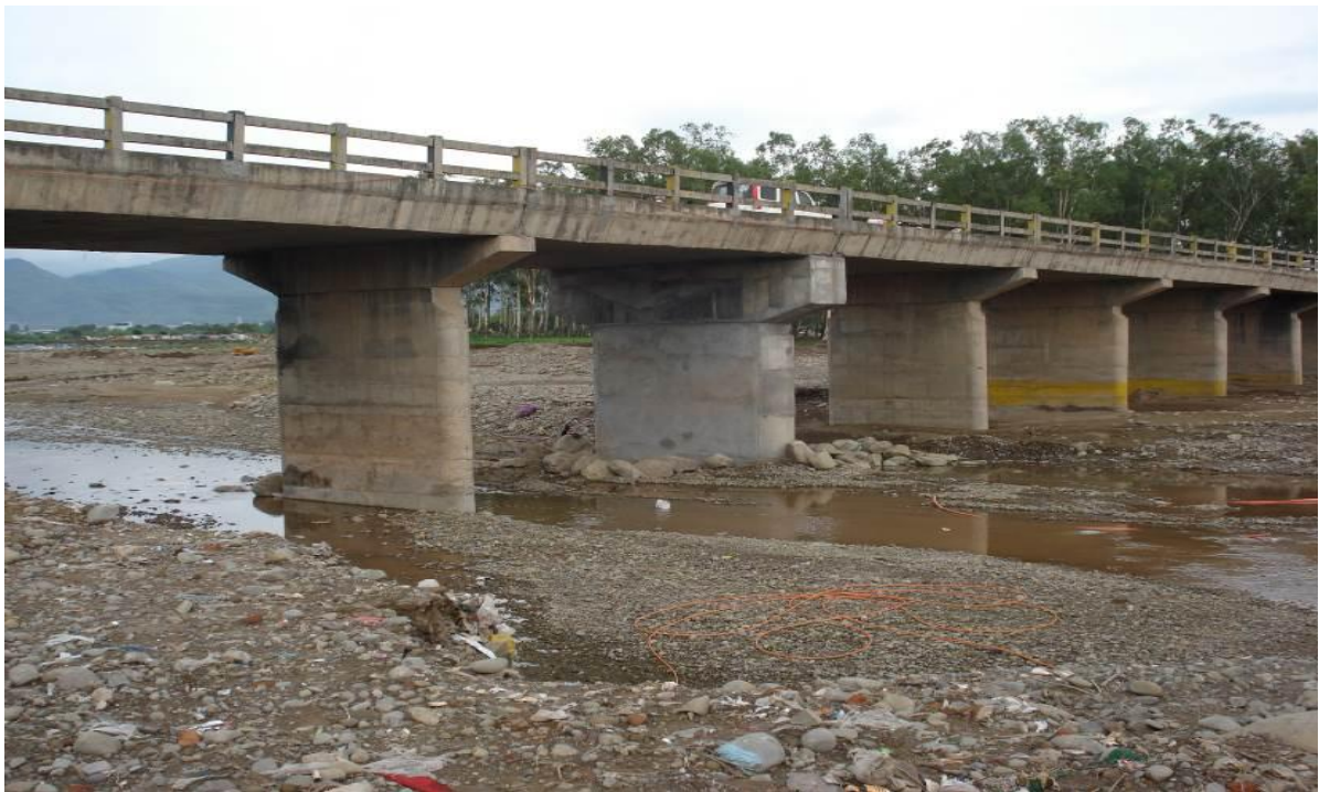
Photo.21. Balad bridge after completion of the rehabilitation works
