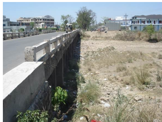
Photo.16. U/S side of bridge near km52 of NH21A
