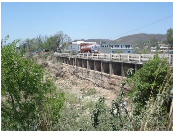
Photo.15. D/S side of bridge near km52 of NH21A
