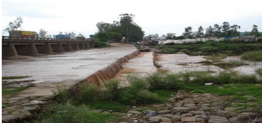
Photo.8. D/S side of bridge near km15 of NH21A
