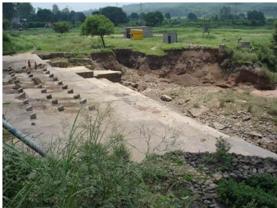
Photo.9. D/S side of bridge near km24 of NH21A
