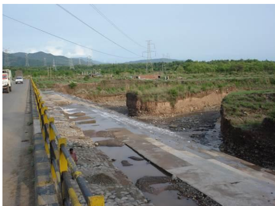
Photo.11. D/S side of bridge near km44 of NH21A
