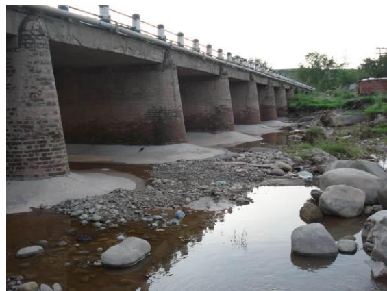
Photo.7. U/S side of bridge across same river
