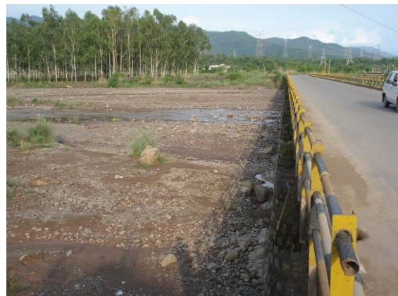
Photo.12. U/S side of bridge near km44 of NH21A
