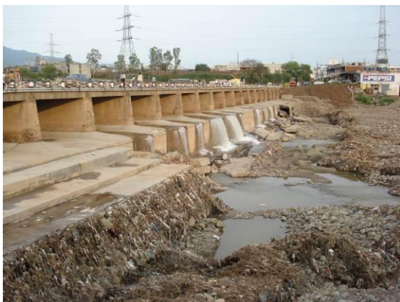
Photo.6. D/S side of bridge across same river
