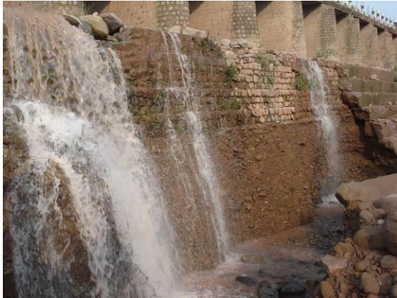
Photo.13. D/S side of bridge near km49 of NH21A
