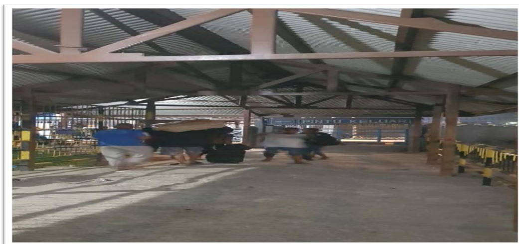
Figure 4. The loading and unloading workers use the descending passenger lane for over-luggage activities Source: PT. Pelindo IV (Persero) Sorong Branch, 2020
