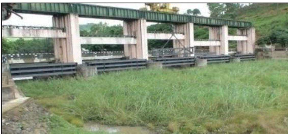
Photo-2: Floating grass (*Phumdis*) deposited in front of the Barrage
