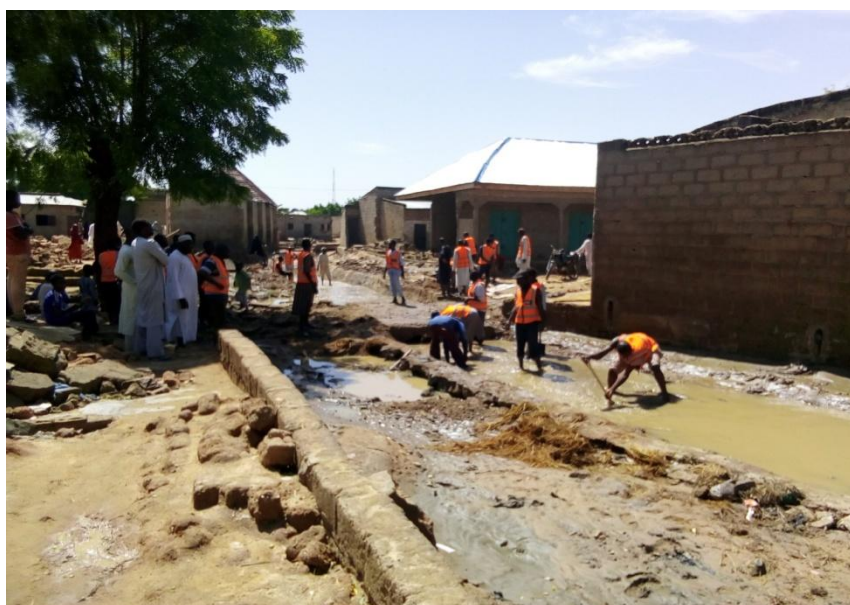
Fig. 3: Some members of IMN carrying out clearance of drainage to permit free flow of rain water
