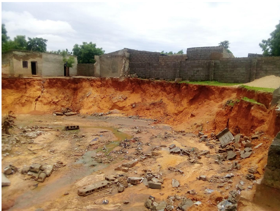
Figure 5: The spot where four houses collapsed and were washed away by the flood waters on July 15 th 2020.
