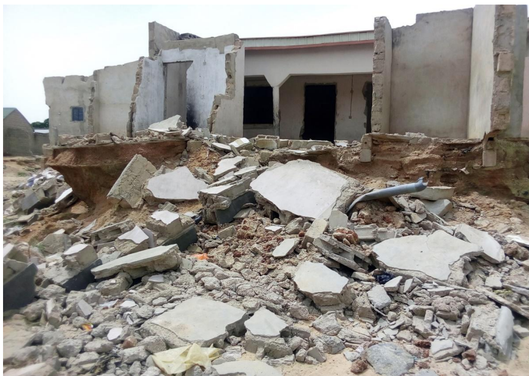
Figure 2: One of the many houses damaged by the flood disaster at Dan Tudu.
