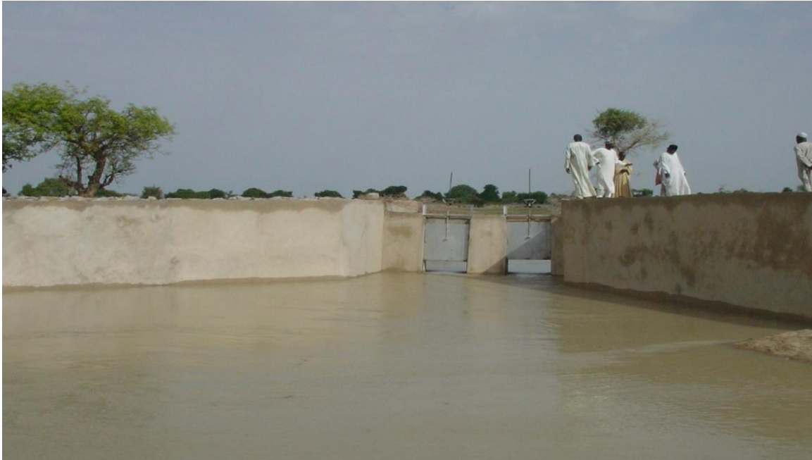
Plate. 1: HJKYB-TFs Double Valve Flood Retention Gate at Kalgeri, Geidam LGA, Yobe State
