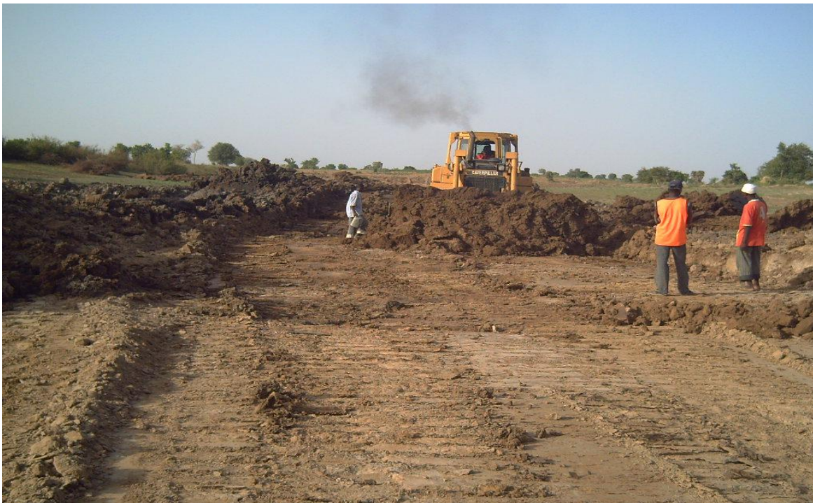
Fig.4a: Channel Clearance in Progress at Kisingin, Kafin Hausa LGA, Jigawa State
