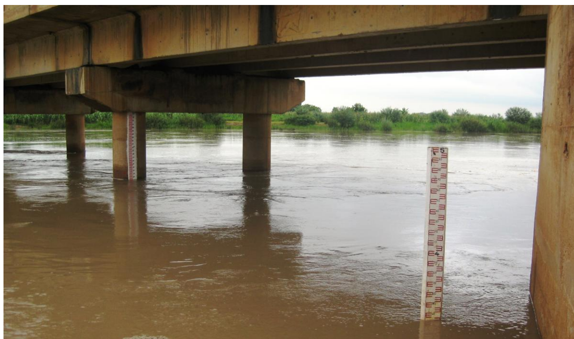
River Gauging Stage Board at Jama'are Bridge Bauchi State
