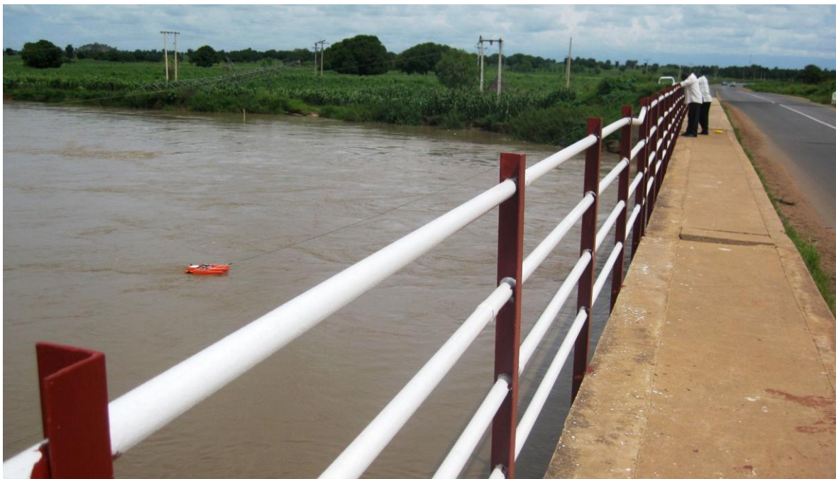
River Flow Measurement using ADCP flow meter at Gwaram Bridge, Jigawa State
