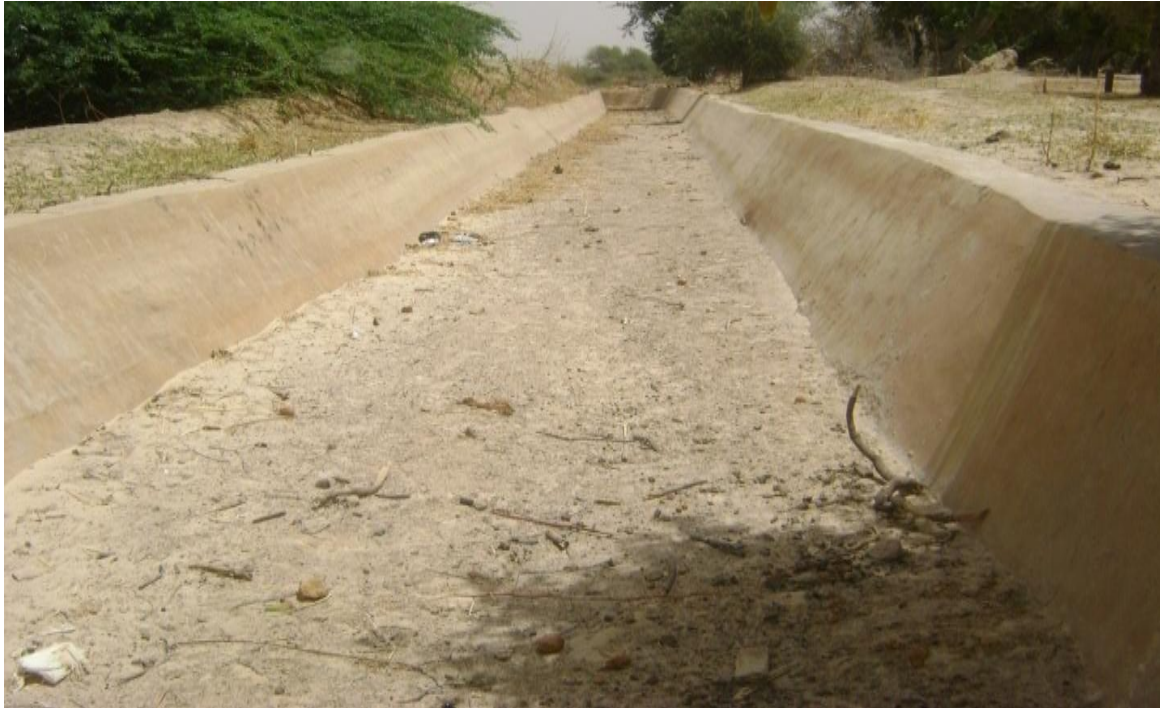
Fig. 3: Concrete Lined Channel at Kanamma, Geidam LGA, Yobe State
