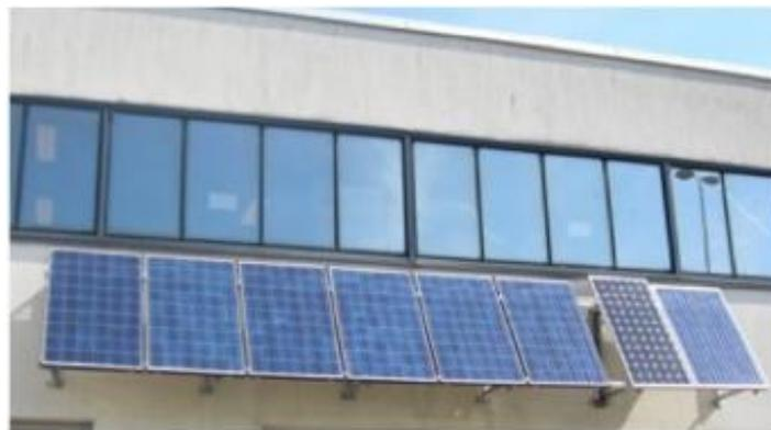
**Figure 2.** Polycrystalline photovoltaic string of 1kWp
