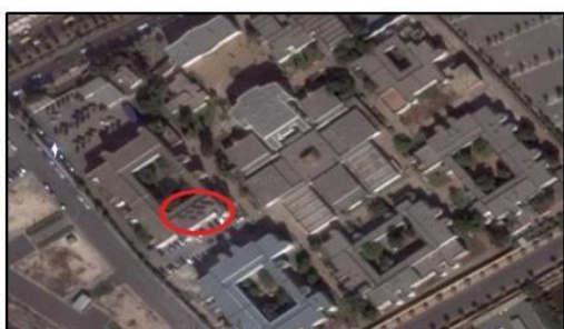
Figure1: .Location of roof by Google Earth.
