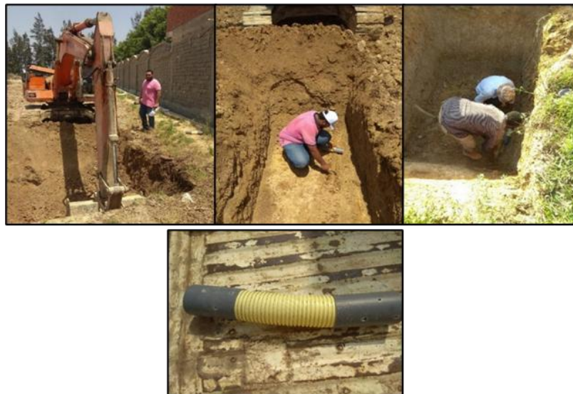
Figure 10. Excavation, sampling, replacing processes, and the two-side coupler pipe
