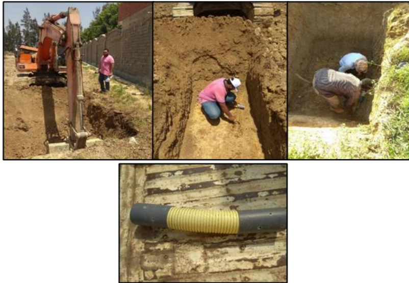
Figure 10 clarifies the processes of excavation, sampling, and replacing the cut section with the new one.
