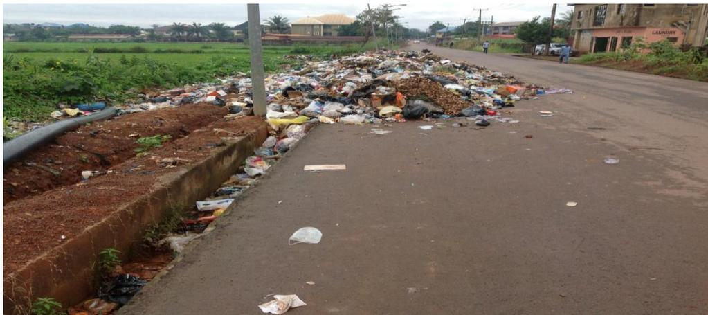
**Figure 3: Blocked water ways due to indiscriminating dumping of waste at Nnorom Street ACT.**
