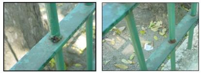
Figures 7, 8 - Aspect in grating corrosion of carbon steel coated with green paint.
