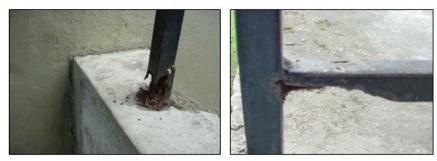
Figures 13, 14 – Appearance of atmospheric corrosion of carbon steel rods.
