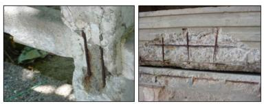
Figures 11, 12 – Appearance of corrosion of concrete by showing the attack on carbon steel by environmental conditions.
