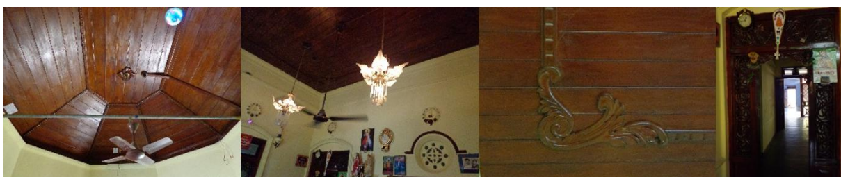
Fig. 5. Ornamentations in false ceiling and doors.
