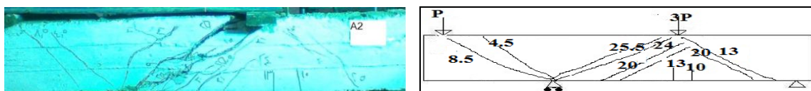
Fig (13) Crack pattern of beam (A2)
