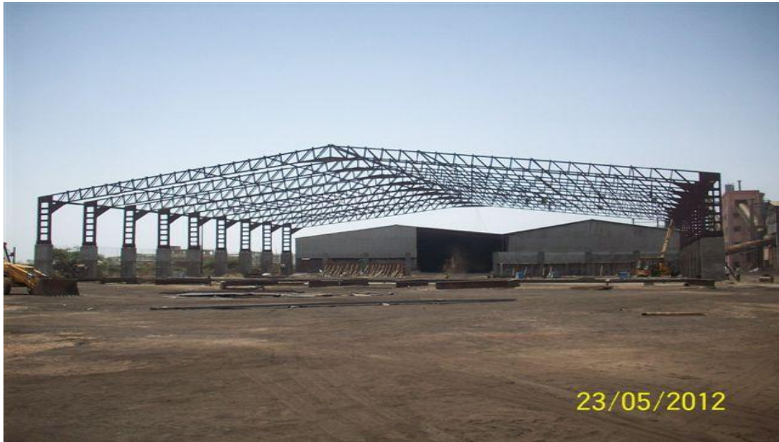
Figure: 1 Lattice Frame Assembly for Large Span
