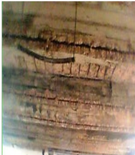
Fig 5c: Exposed reinforcement in slab and beams
