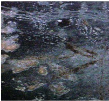
Fig. 5a: Spalled concrete surface
