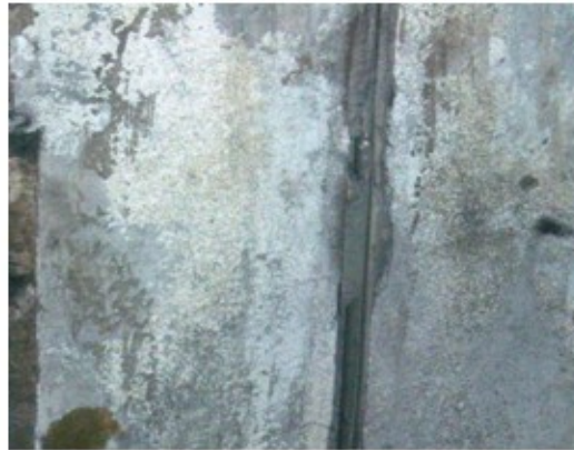
Fig. 5b: Blemished concrete surface
