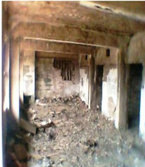
Fig. 5d: Delaminated slabs, beams and columns
