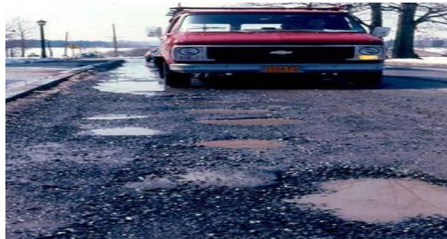
**Fig 10. Potholes caused by poor drainage**
