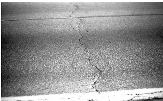
**Figure 5. Low severity transverse crack.**
