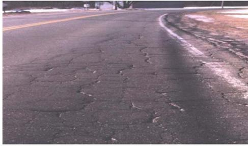
**Fig 3. High severity alligator cracking**
