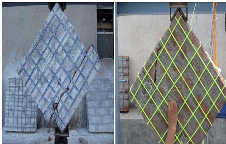
Figure 3-Failure of panel retrofitted with (a) Polypropylene Strips (b) Nylon Wire
