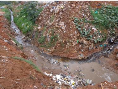
Figure: 5 Unobstructed Leachate flow as well as stormwater at the Leachate Collection Sump - September 2013
