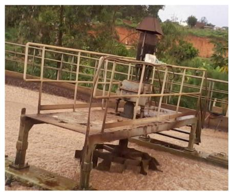
Figure:4 Aerator B with signs of corrosion
