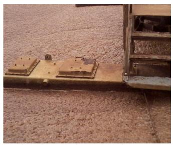
Figure: 3 Corroding floater and stairs for Aerator C
