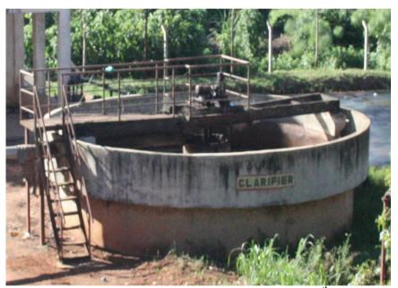
Figure: 2 Clarifier stairs and dilapidated center support 30<sup>th</sup>Nov 2013
