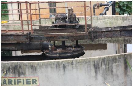
Figure: 1 Clarifier center support photo taken on 30th Nov. 2013.
