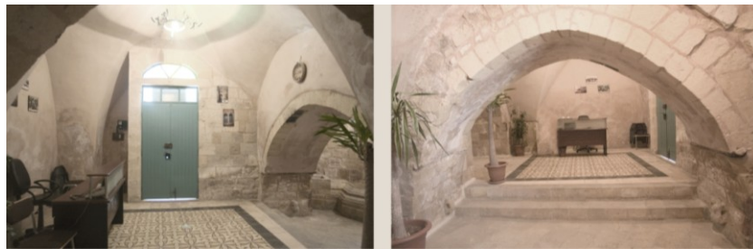
Fig. 11 Madafat Farah Abu Jaber one main barrel vaulted gallery leading to other cross vaulted rooms. Source: Author 2013
