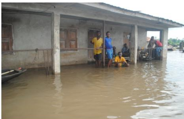
The picture above shows a house flooded at Odeke Ibaji during flood disaster.
