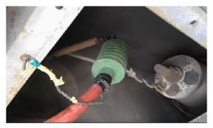
High Tension Cable connected to the Field of E.S.P
