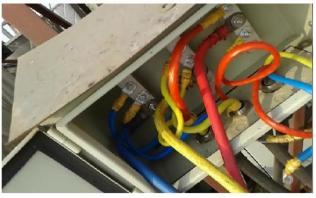
Three phase supply connected to the Transfomer
