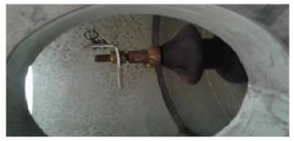
Transformer Bushing(supply is connected to Transfomer Bushing
