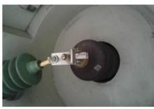
ligh tension Cable connected to Transformer Bushing
