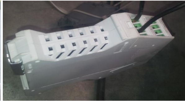
Fig.15 Converter installation at the site
