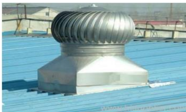
Figure.1. Roof Top Ventilator
