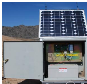
b) Sink node in a cabin
