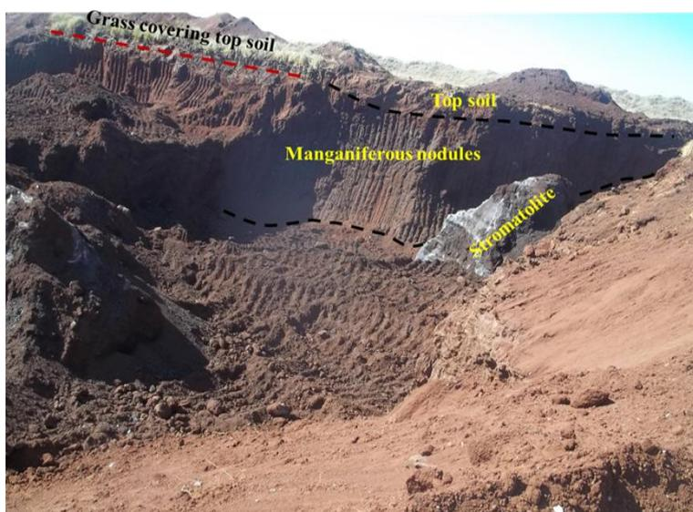
**Figure 4:** An open exploration borehole showing the profile setting in the mine area. GPS coordinates (S 26° 8' 5.8"; E 27° 15' 32" and elevation: 1554 m).
