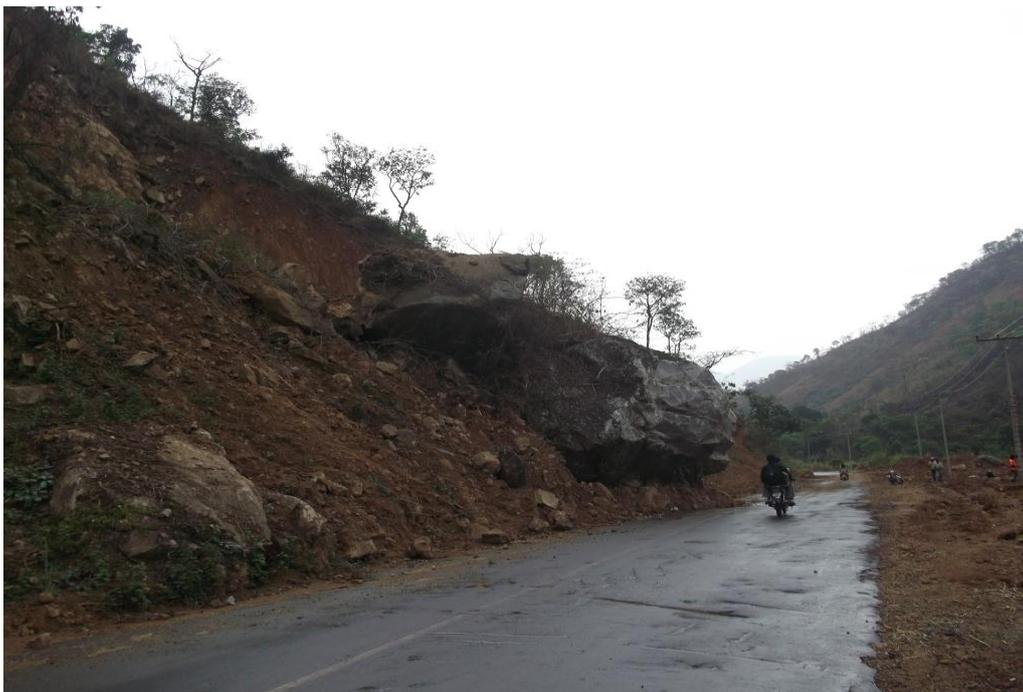
**Fig. 8** Picture of slope OB1, showing the threat posed by this slope instability on road users.
