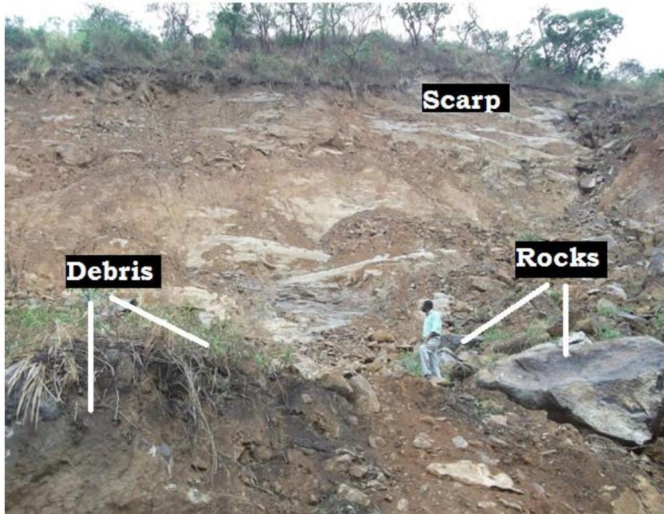
**Fig. 7** Picture of slope OB1 showing the scarp of the slide, as well as the rocks and debris moved.
